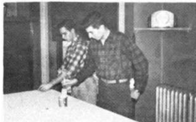
BETA SIGMA "Help Week" demonstrators (William Mann, Carl Krebs, and William Kinhead) install fluorescent lighting at the Blind Association house; Ralph Meerworth, Wells Staub, and Lloyd Painter work on a shuttle bin; Lloyd Painter and Meerworth paint a reconstructed storage bin.
