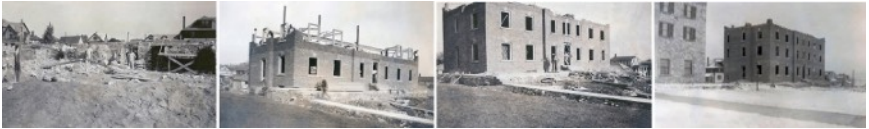
House Construction from September to December 1929
